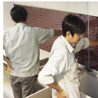
HOLD GLASS IN PLACE FIRMLY approximately 15 minutes for silicone gel to dry.
