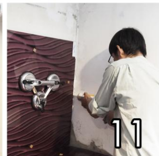
ADDITIONAL SEALANT GEL placed gel around corners and sides of glass to increase adhesiveness.
