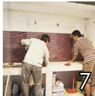
WALL GLASS INSTALLATION meticulously and carefully.
