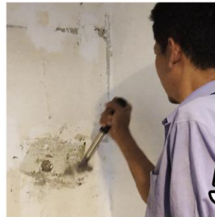
USE WALL SCRAPER to smoothen the wall surface area. Workers to service the wall surface underneath the 3D glass carefully.
