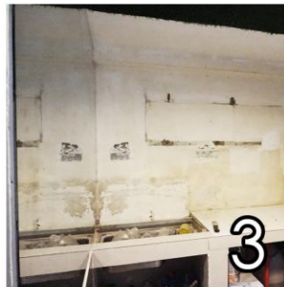
REMOVE items and furniture where 3D glass will be installed.
