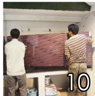
ARRANGE TWO 3D GLASS PANELS carefully so that they are tightly fit.
