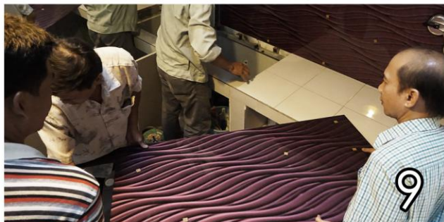
INSTALL SUBSEQUENT PIECE OF GLASS slowly and carefully place the glass in place.
